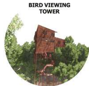
Figure 9. Bird observation/ viewing tower.
