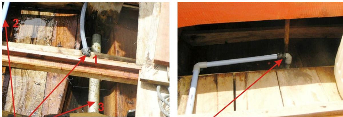
Figure 6. Installation of Motor Drive Tubes and Rubber Pipe.
